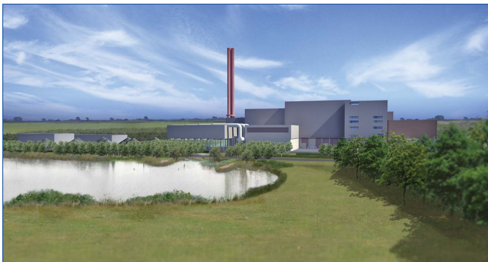
North view of the Resource Recovery Facility
