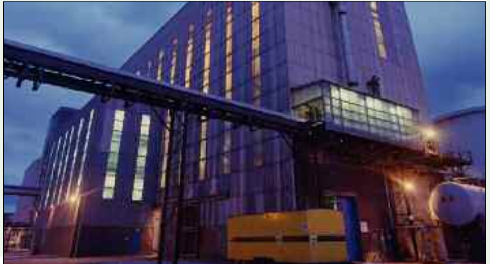
■ British Salt's Middlewich plant
